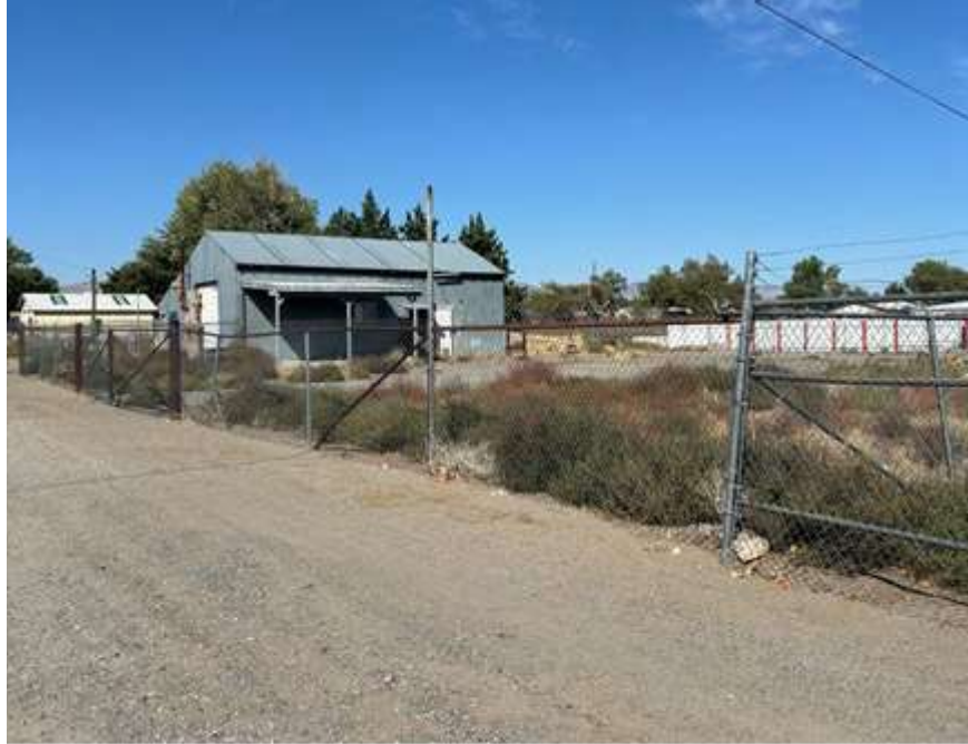
Figure 2: Project site showing vacant portions of the parcel (from Woodchuck Dr facing northwest)
