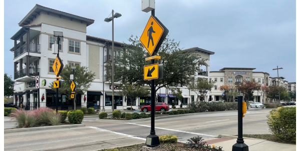
RRFB (Rapid Rectangular Flashing Beacon) and bulb outs to enhance pedestrian safety and increase surrounding aesthetics.
