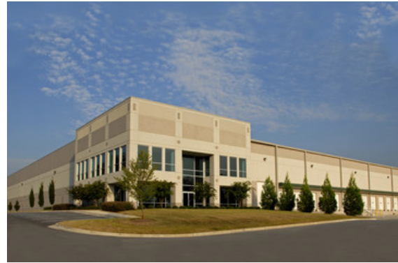
Industrial building with horizontal/vertical stepbacks.
