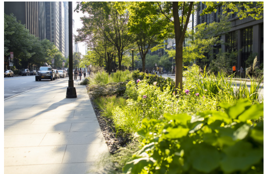
Bio-retention basin to treat stormwater runoff and enhance streetscape.
