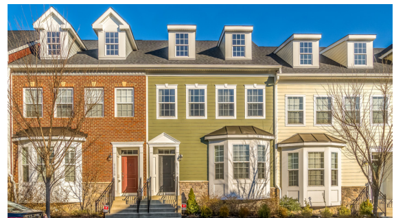
Townhomes with sidewalk access to active street frontage.
