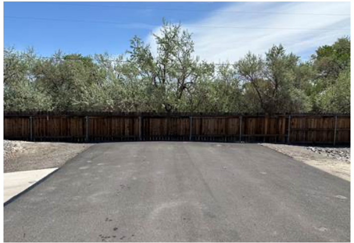
Access from Quick Cal Way
