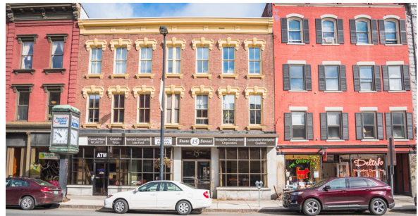
Slight variations in building heights and roof profile with on-street parking.
