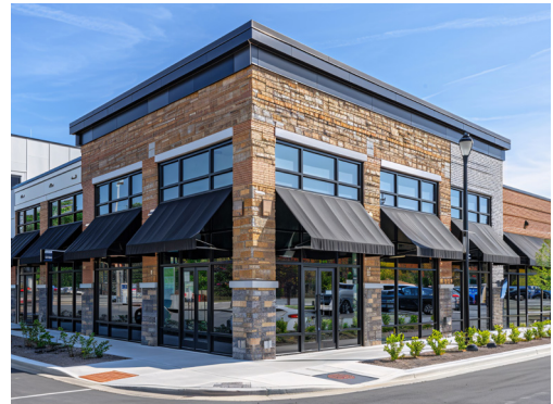
Variations in building facade and articulation.
