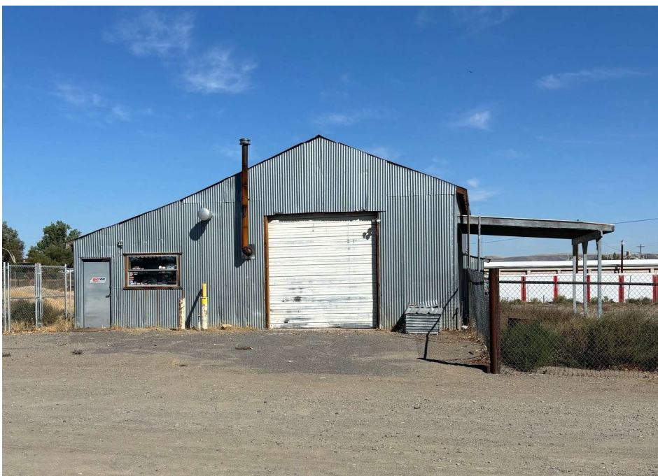
Figure 1: Existing commercial structure (from Woodchuck Dr facing north)
