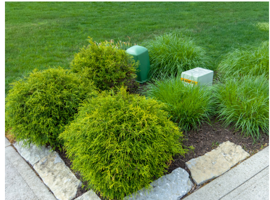
Landscaped screening of utilities
