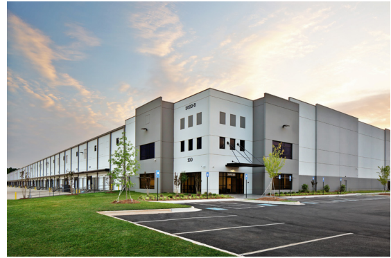
Parking located around the perimeter of the site.
