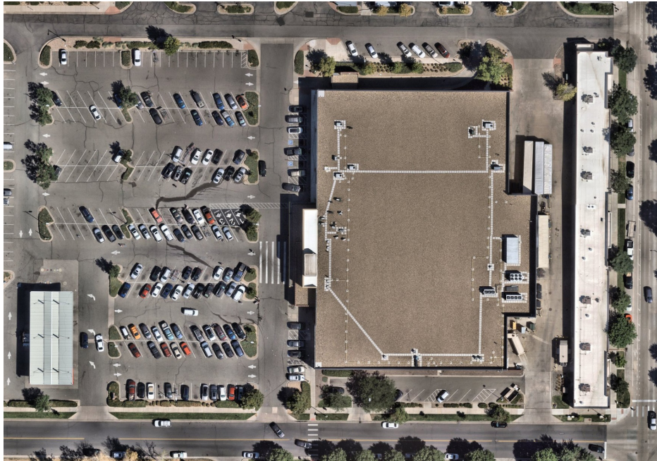
Shared loading area located at the rear of the building.
