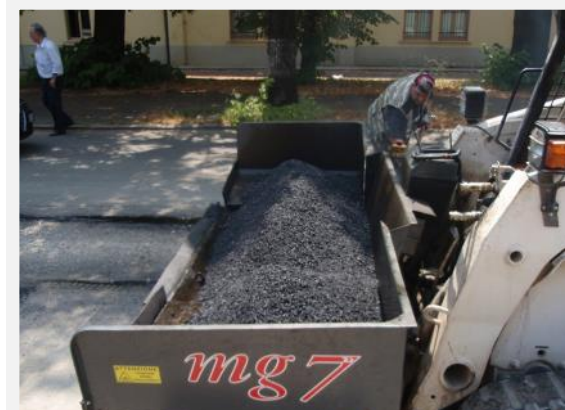
MG7 paving a shoulder.
