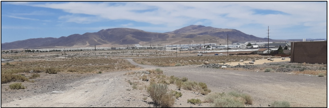
Overall site – view north
