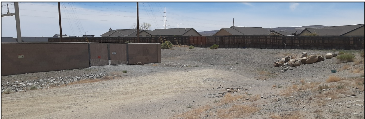
NV Energy substation panorama – view southeast
