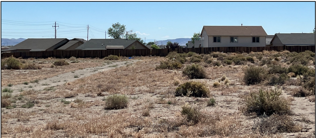
Houses on east boundary – view north-northeast
