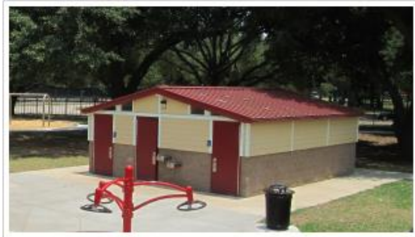
Image 6: ADA-Compliant Standalone Modular Restroom Facility
