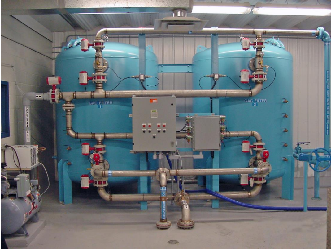
Figure 4.6 Photo of parallel/series pressure vessel pair
