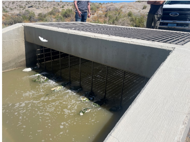
b) Outfall Channel and Screen
