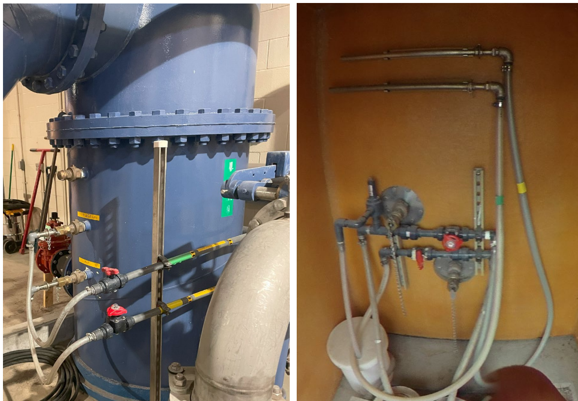
FIGURE 2-5: TREATED WATER CAUSTIC SODA DOSING POINTS TO PERMEATE (LEFT) AND FINISHED WATER (RIGHT)
